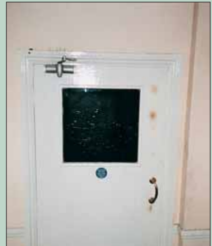
Wired glass is often used in exit doors, such as this one.
