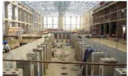
Sejal's new float line will produce 606 tons of glass per day.
