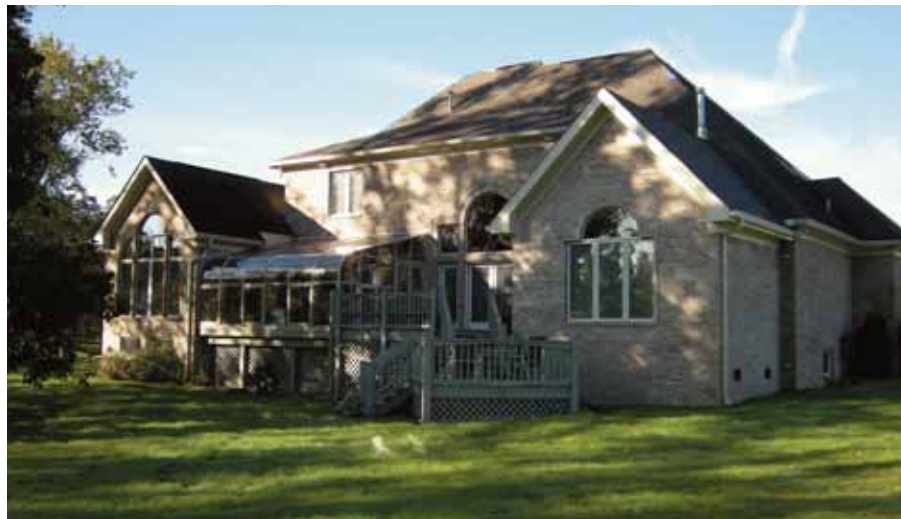
This sunroom provided by Four Seasons Sunrooms won in the category of Glazed Roof Sunrooms $35,000-$50,000.
